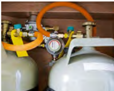
„Truma Duo Control CS“ gas regulation system
